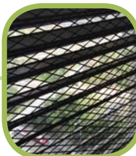
Louvred corridors facilitate natural ventilation to reduce dependence on air-conditioning.
