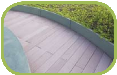
The roof decking is made from recycled plastic and wood waste. 天台地台板以回收塑料和木屑合製而成。
